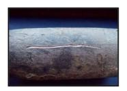
Lead service lines are generally a dull gray color and are very soft. You can identify them easily by carefully scratching with a key. If the pipe is made of lead, the area you've scratched will turn a bright silver color.
